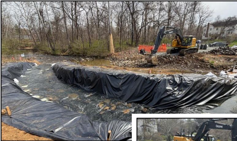
Installation of water diversion
