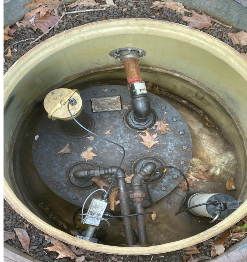
Overview of Tank
