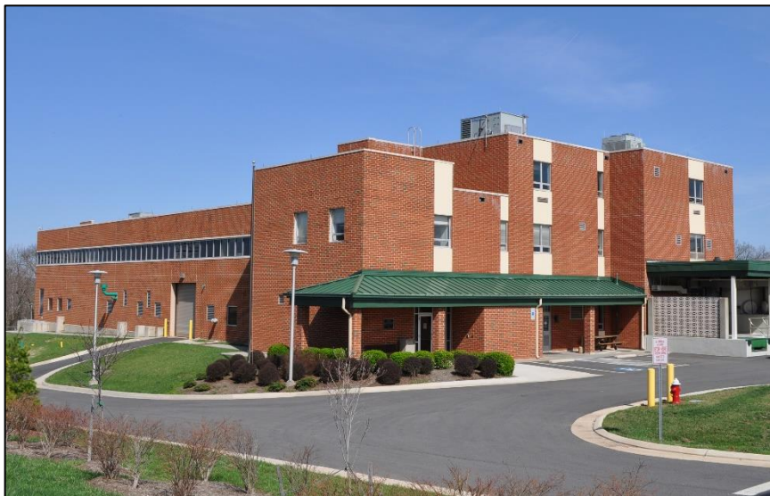
Kenneth B. Rollins Water Filtration Plant
