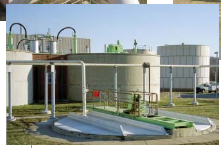
Odor Control Covers at Gravity Thickener
