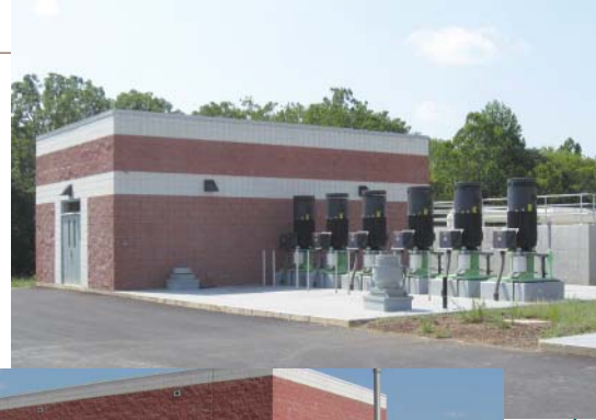
Effluent Pump Station
