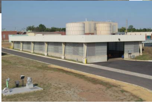
Soil Amendment Storage Building
