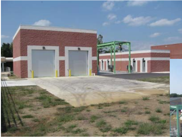
Influent Pump Station Screening Room
