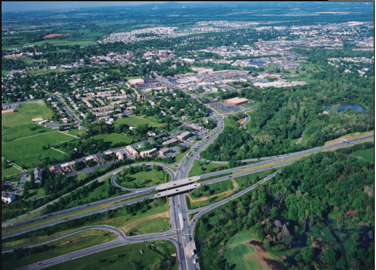
"The Town of Leesburg in Virginia" looking north at intersection of King Street (U.S. Route 15) and the Route 7 and 15 bypass
