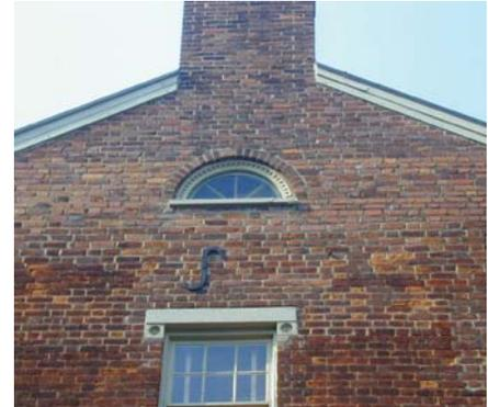
Brick structures should be inspected regularly for signs of weather or moisture-related deterioration. Older brick may lose its hard outer surface leaving it vulnerable to moisture penetration. Mortar joints may crack or erode, allowing another avenue for moisture to enter an exterior wall.
