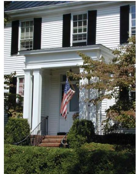
Well-maintained, wood-clad frame structures may last indefinitely. Paint should be inspected for condition on a regular schedule as its condition may be the first warning signs of a moisture problem within the structure. Any junction between elements, such as between siding and window trim, should also be checked for soundness.
